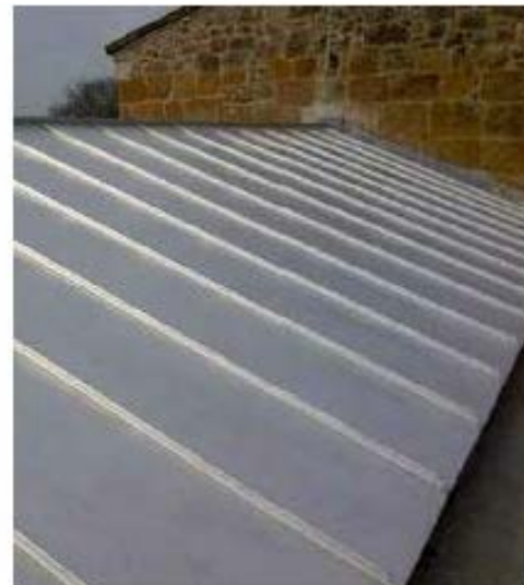
Standing seam metal roof
