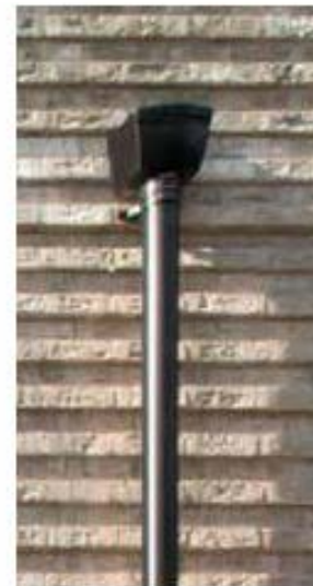
Rainwater pipes replaced
